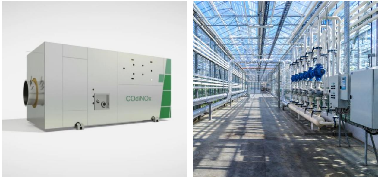
Figure 10.5. Exhaust scrubber (left) and CO 2 piped into the CEA facility after scrubbing (right) Source: Hug Engineering (n.d.)
