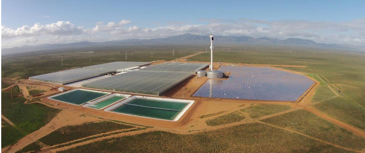
Figure 5.5. Solar thermal at a CEA facility
