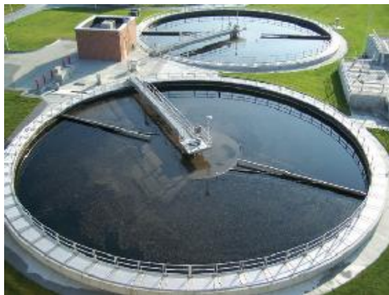
Figure 7: Example primary clarifiers.
